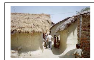
Design consideration and regulatory framework can help reduce fire hazard in such settlements and improve housing quality
