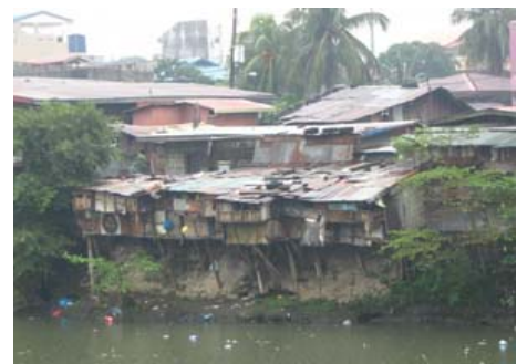
Figure 5. Informal settlement along banks of San Juan River at the back of CCP.
