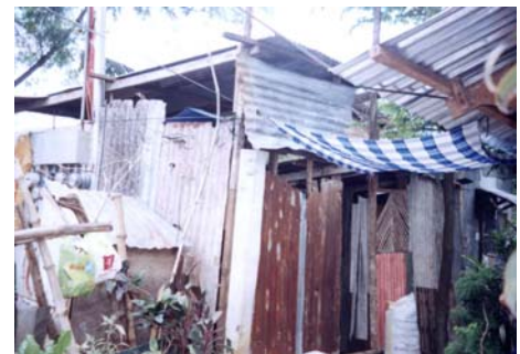
Figure 2 Building materials in an informal house show the use of galvanized iron sheets for both roofing and walls.
