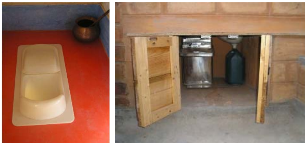
Tin drum for faeces and barrel for urine collection
