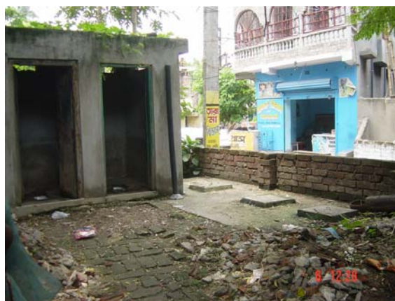
Position of tubewell and septic tank - 2
