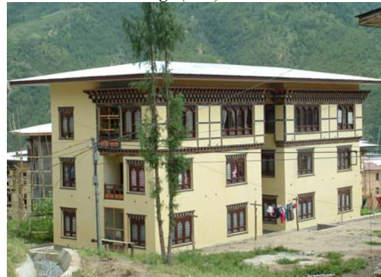
II Buildings (new)
