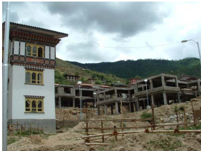
Construction of phase III Buildings
