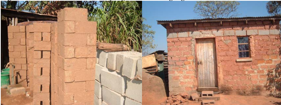
Figure 4 Concrete and earth blocks for grade II building regulations
