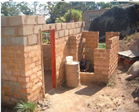
Figure 9 Building construction going on
